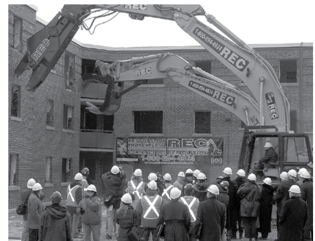
detail, demolition, 2006. © Dagda
