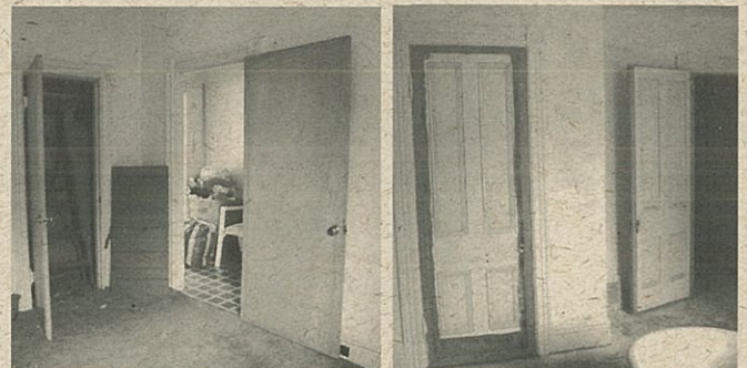
The original pine doors, encased in plywood covering, are revealed.
