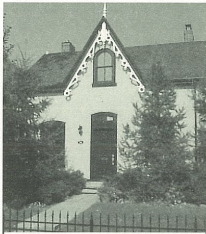
One of our wonderful restored Amelia Street Cottages
