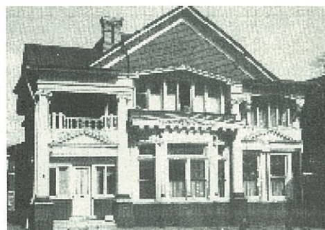
1982—showing the west façade.
